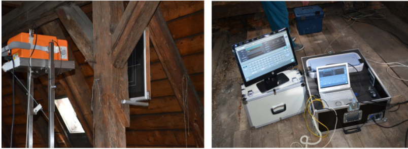
Fig. 9: Experimental device for monitoring building elements.
